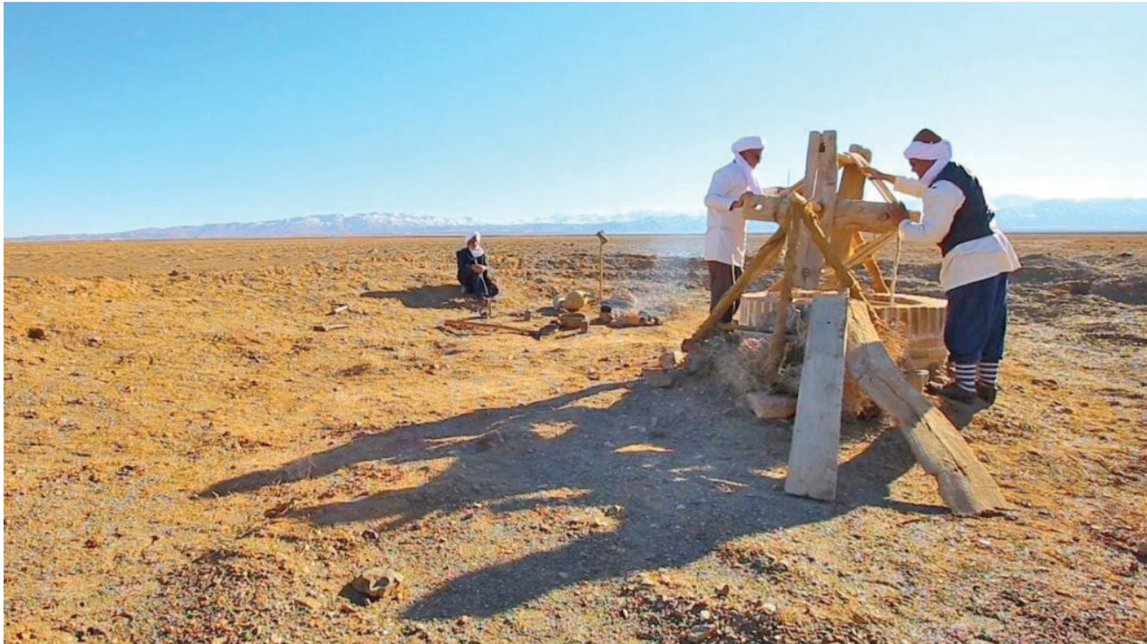
Qanat is a gently sloping subterranean canal, which taps a water-bearing zone at a higher elevation than cultivated lands.
