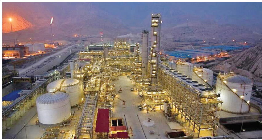
Karoun Oil Cluster power plant.
