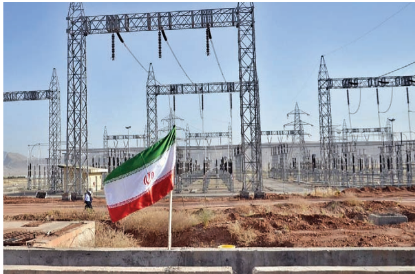
of 28 electricity distribution lines, increasing Gorgan transmission substation capacity, as well as improvement and optimization of stations, transmission lines, and water
