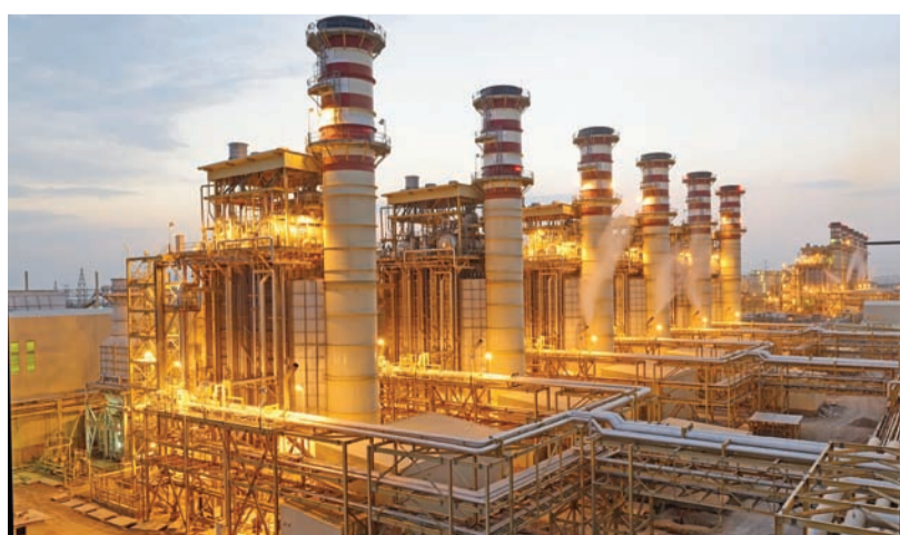
Damavand Combined Cycle Power Plant
