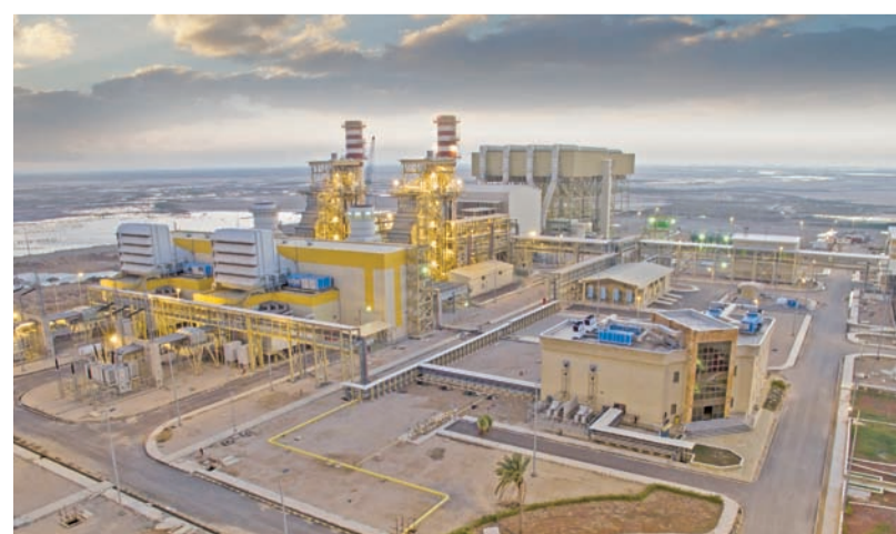
MAPNA Genaveh Combined Cycle Power Plant 2
